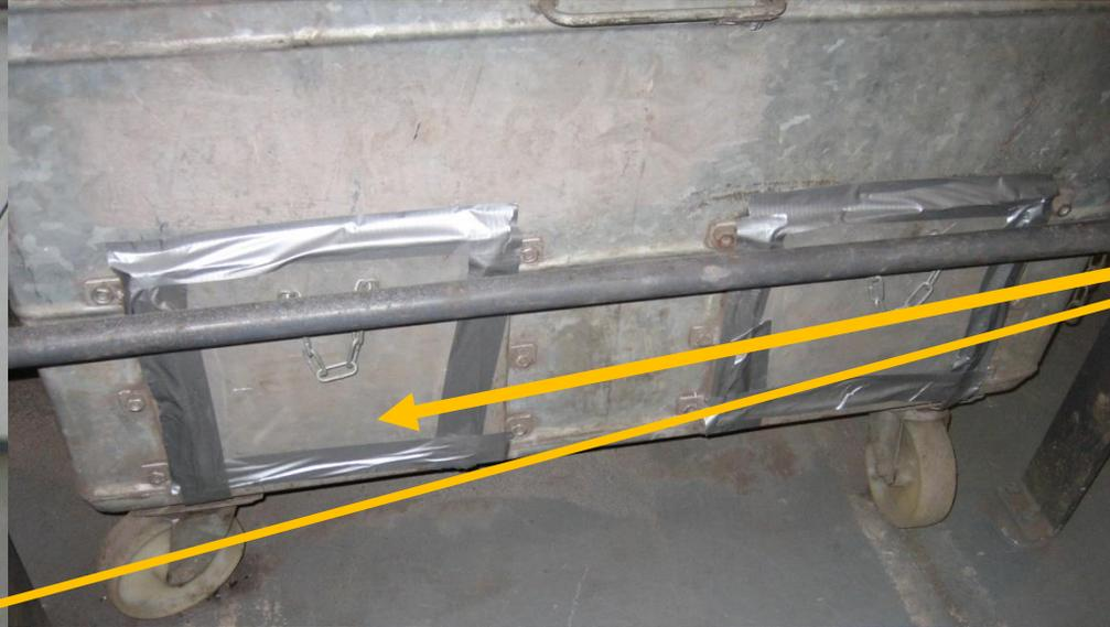
Ash bin doors modification can allow false air into the boiler
