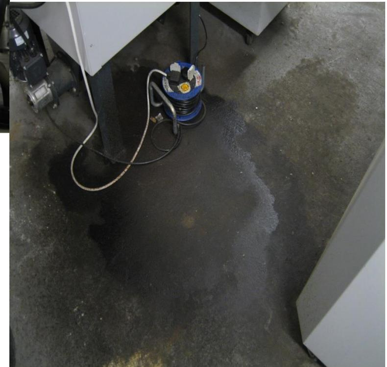
A combination of some simple boiler faults, a power cut, BMS inconsistencies and extended repair response times result in a dirty floor and lost R.H.I. revenue.
